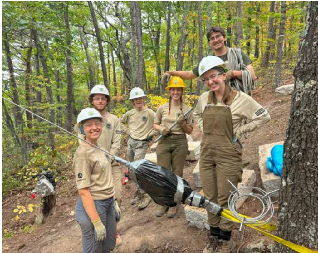
Photos, top left: Members of the Appalachian Conservation Corps stand behind the highline hoist used to move 600 pound granite steps.
